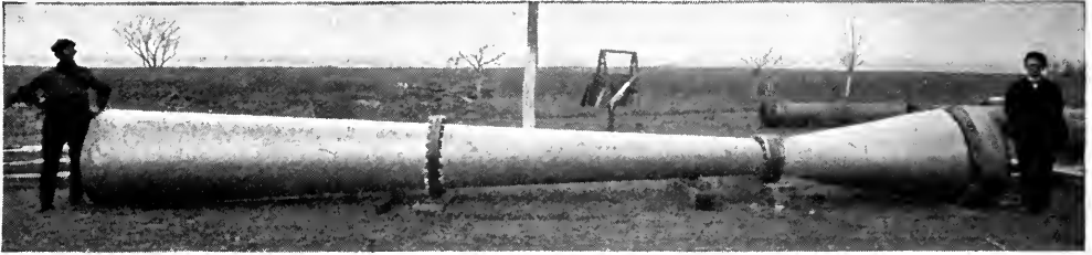
METER TUBE BEFORE INSTALLATION AT PUMPING STATION
